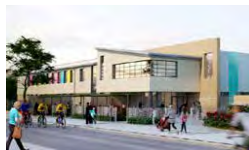
Northstowe primary school, as part of the street scene
